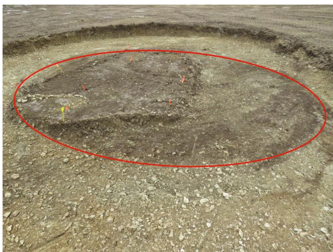
Fig 10-1, USBC-002, filled in the crater in the dark area, WWIIBRPG
